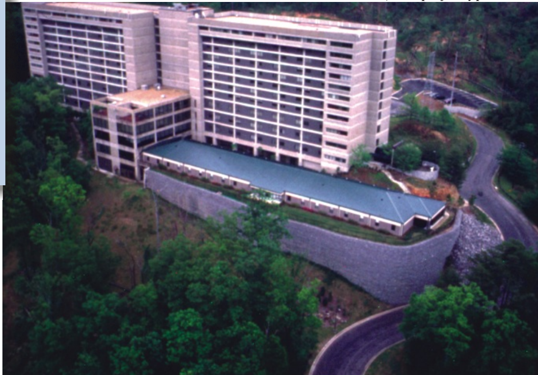
MSE Wall in Vestavia Hills, AL. Specified by private owner.
